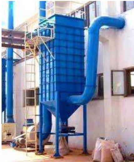
Pulse Jet Type dust Collector
